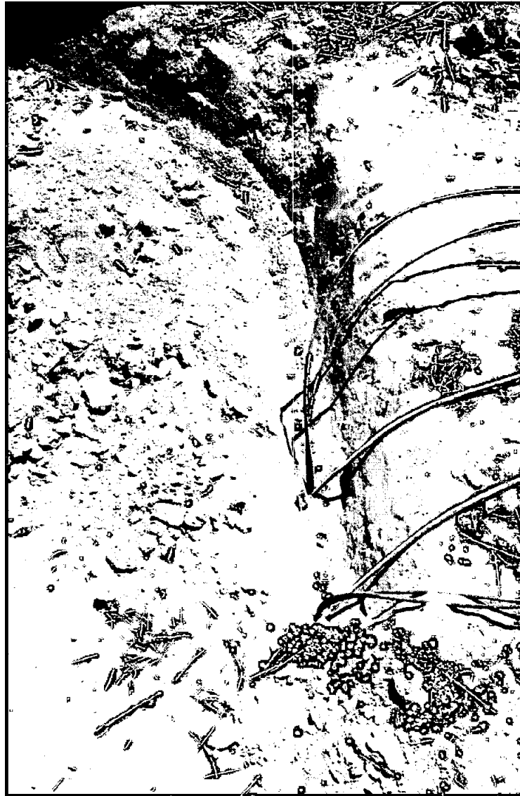
Figure 10. Trench dug to bury cables and tubes.
